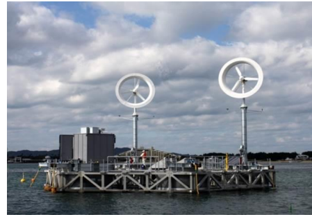
Fig.4. 18m wide concrete platform of offshore hybrid floating energy farm by Kyushu Univ. at Hakata-bay, Japan
